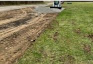
Laid out and painted parking out sod and installed gravel for new parking lot
